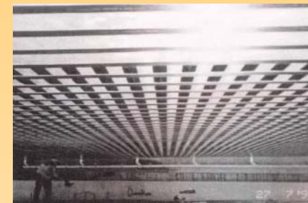
Applied CarboDur CFRP Plates
